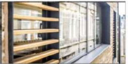
Example of: Timber Bris Soleil (Photograph indicative) Actual colour and fitting to be confirmed. Timber Bris soleil to be installed to south facing classroom windows with horizontal profile and PPC support frame.
