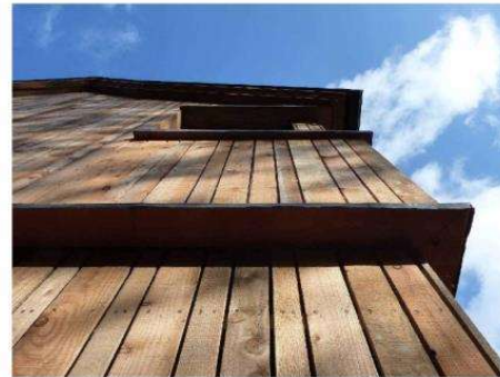
2. Random width Larch timber cladding
